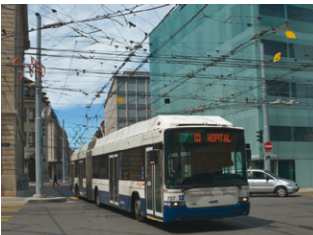
Figure 6.1: Trolleybus infrastructure (photos by Per Gunnar Andersson)
