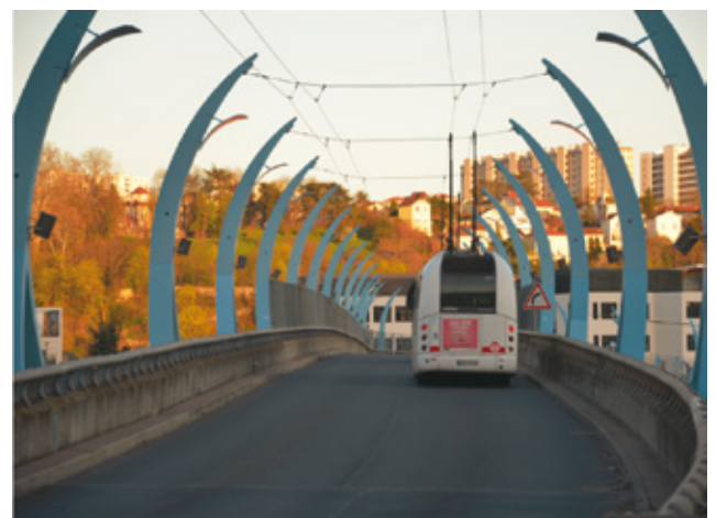
Figure 6.2: Trolleybus infrastructure (photos by Per Gunnar Andersson)
